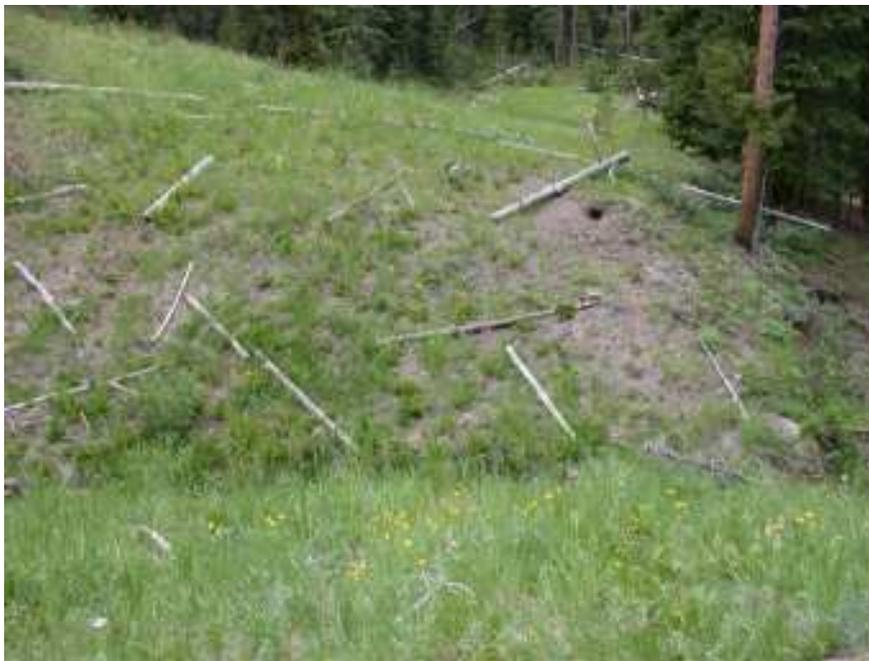
**Photo 7. East Fork FK Cache Ck Road.** The road surface was ripped, seeded, and drained. Logs were placed on cutbank slope to catch sediment and stabilize the slope.
