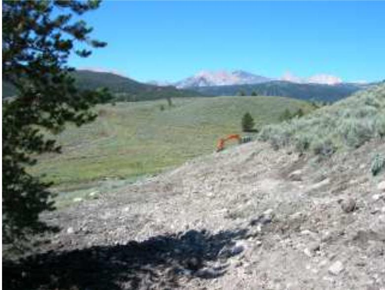
**Photo 4 . Re-contoured road in T9S R3E S1.** Treatment consisted of pulling fill slopes and packing back in the road prism to cover the cut slopes. Topsoil was placed on the surface as much as possible. The re-contoured road prisms were then seeded and hydro-mulched. The upper left part of the picture is a road segment to a former cabin which was ripped, drained, and seeded (Photo taken on 7/27/05).
