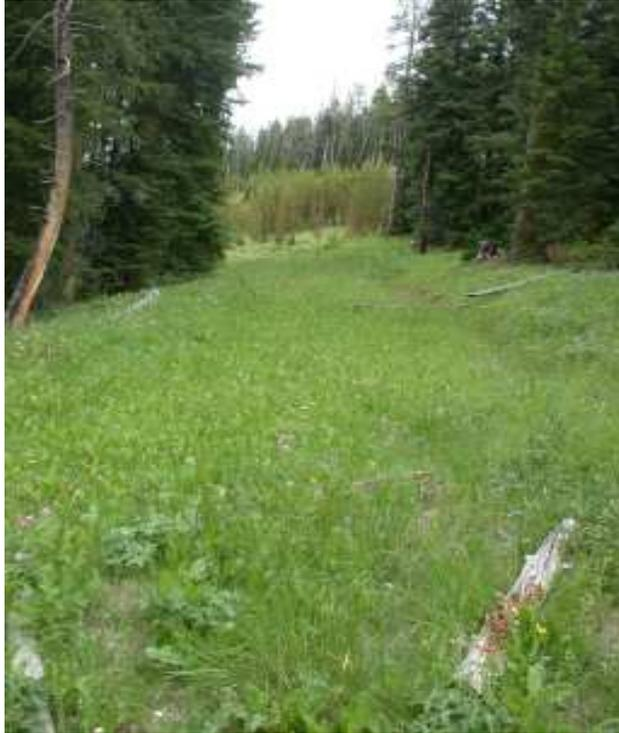
**Photo 8. East Fork Cache Creek Cache Ck Road.** Seeded and Stabilized Road. This road section is typical of most of the decommissioned road segments in Cache Creek. Note lodgepole regeneration in historical timber harvest unit in the distance. Both the road and timber harvest unit in this area are no longer sediment sources to Cache Creek.
