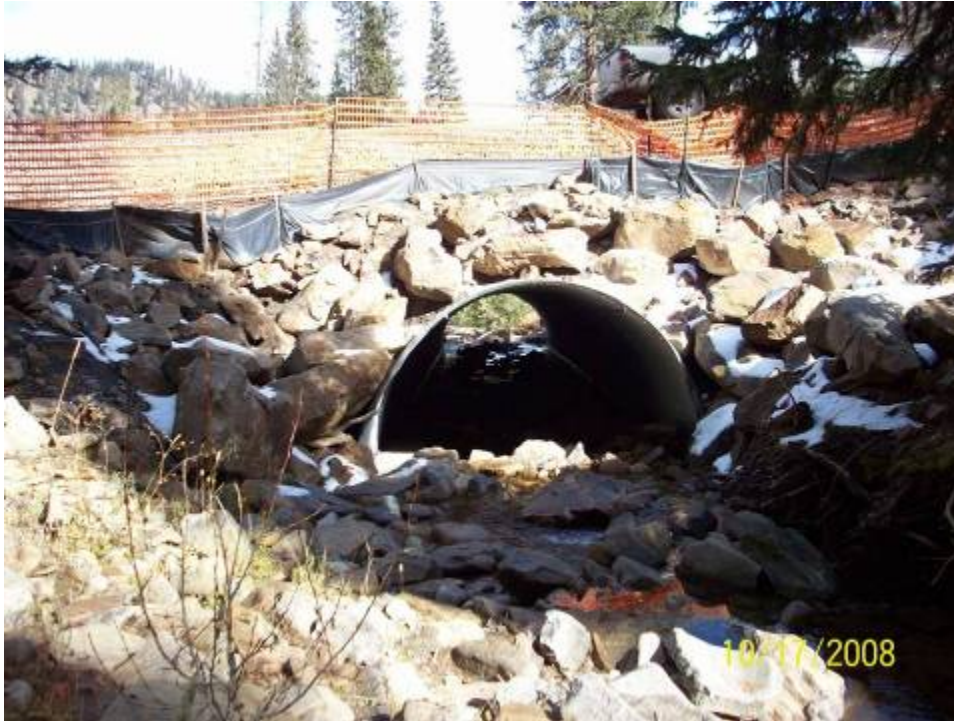
Photo 5. Silt fence installed at road crossing.
