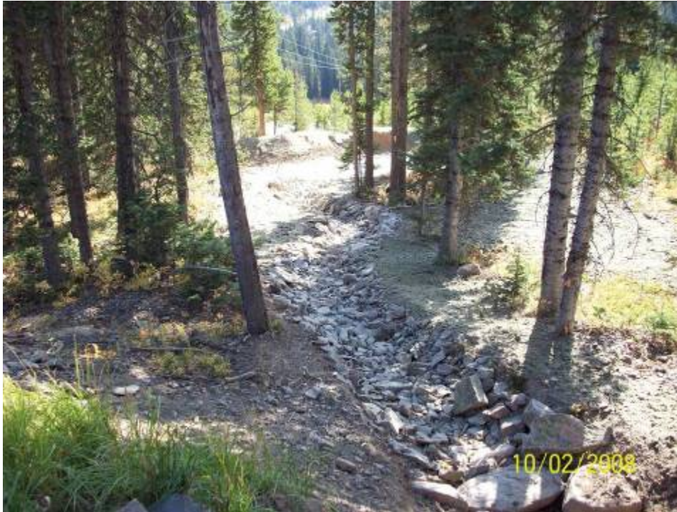
Photo 3. Rock lined storm water conveyance channel.
