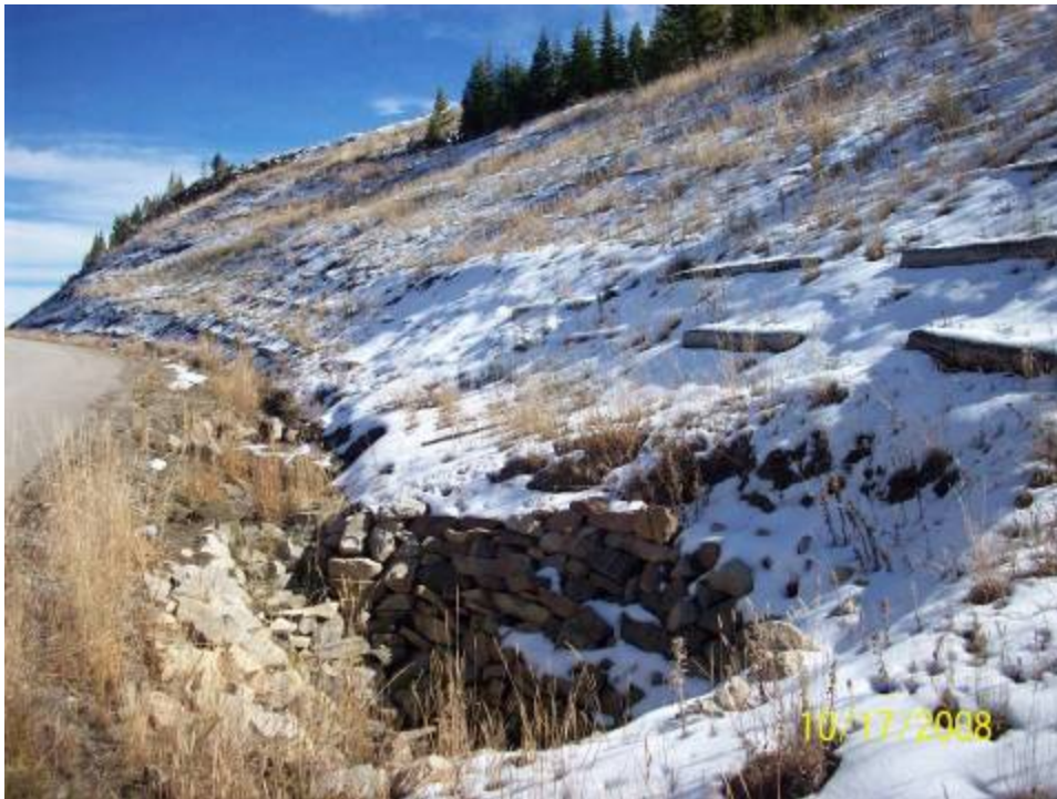
Photo 6. Hillslope terracing with logs and inlet protection at culvert.
