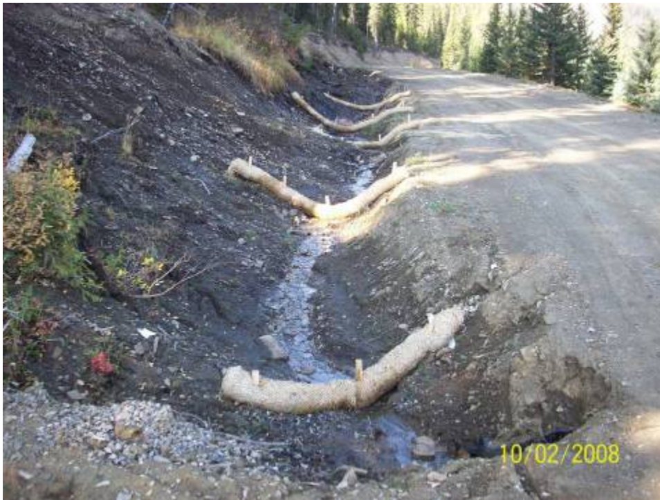
Photo 2. Fiber wattles used along a road ditch.
