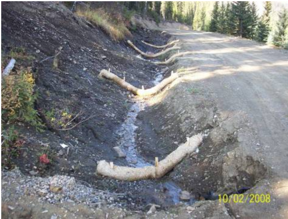
Fiber wattles used to control road ditch erosion.
