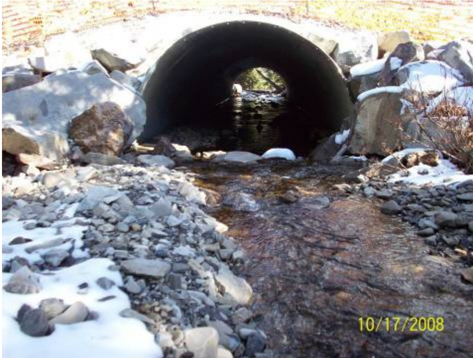
Bottomless corrugated steel culvert.
