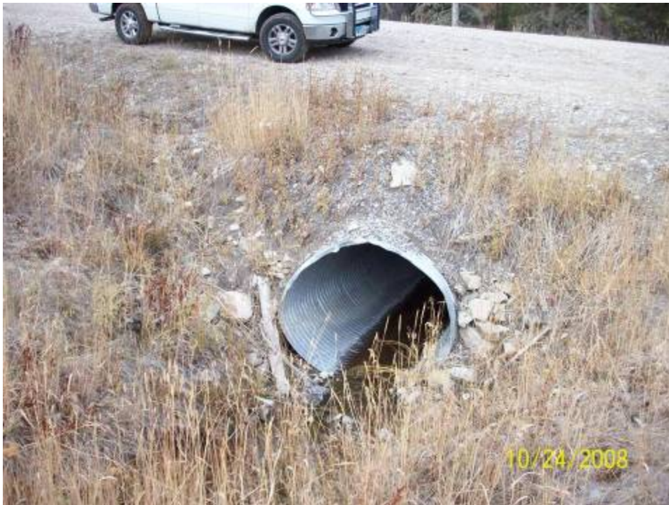
Correct culvert installation.
