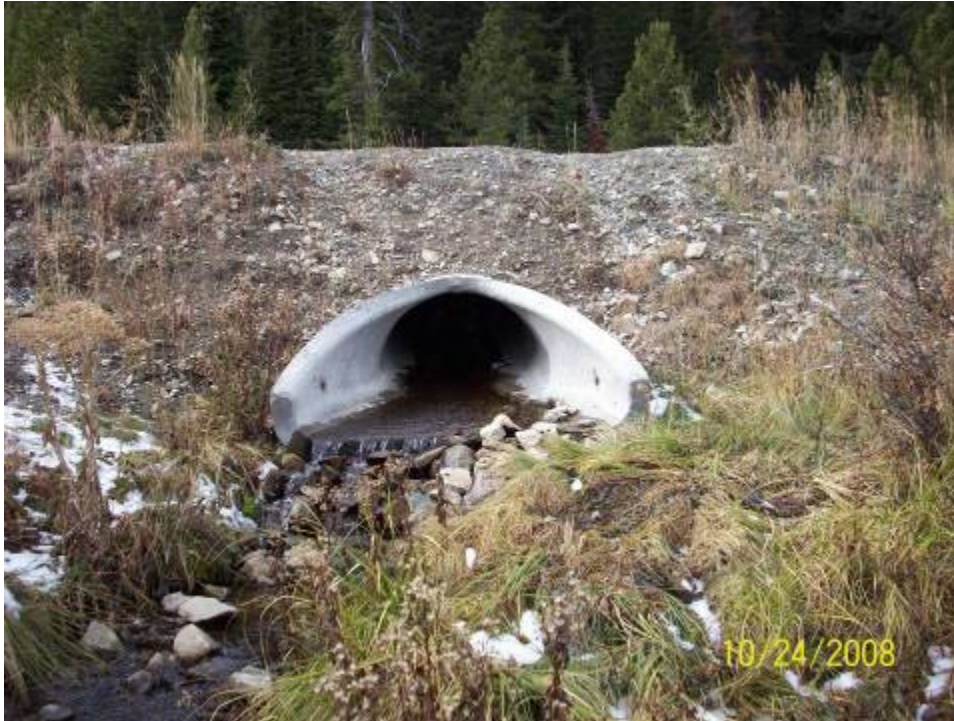
Example of concrete culvert.
